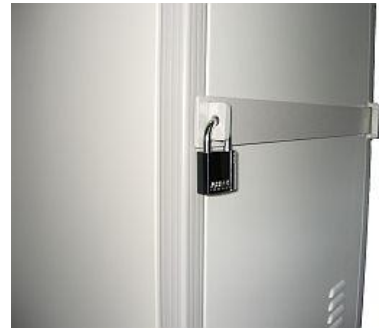
Security Bar & Padlock on Door
