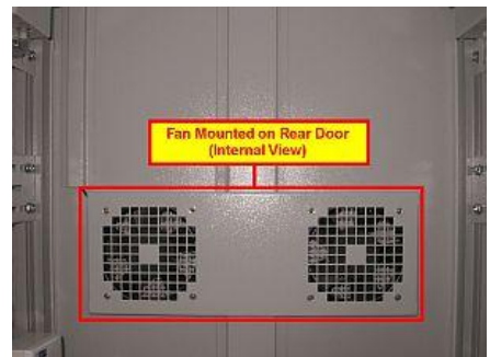
Fan Mounted Louver Rear Door (Internal View)
